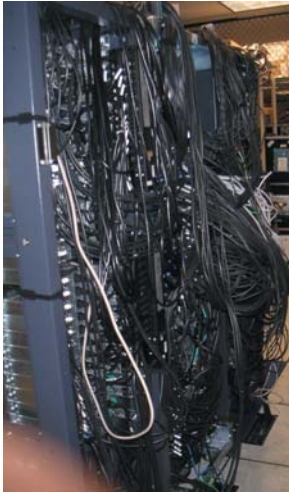
Figure 5: Traditional Cluster Cabling
