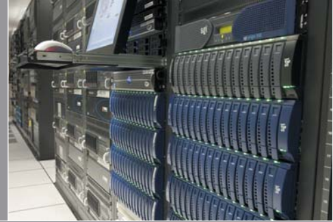
SGI® InfiniteStorage installation at NBA Entertainment
