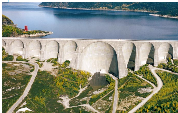
The Manic-Outardes coffer dam
